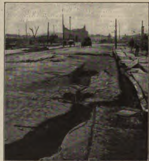
Fissures made by earthquake. (From a photograph.)
